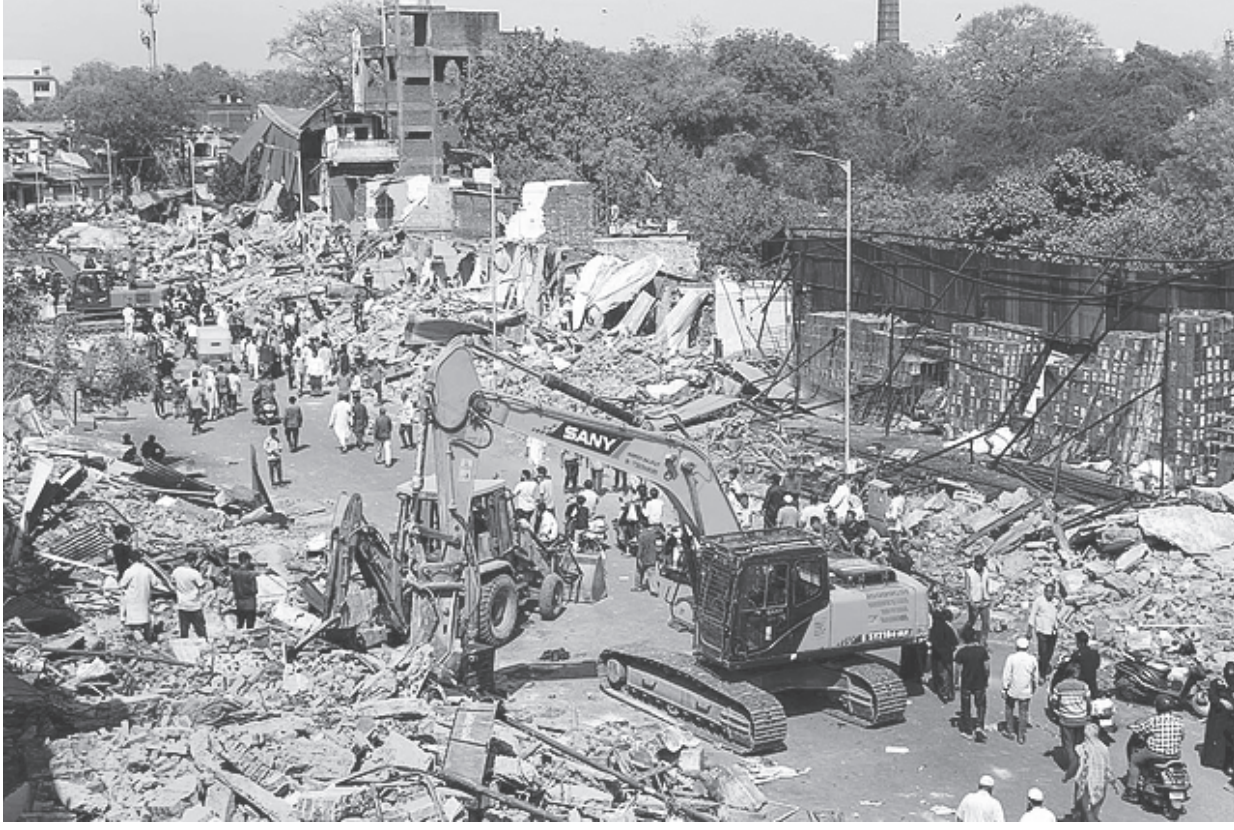
Earthmovers demolish illegal encroachments along a road during an anti-encroachment drive by Ahmedabad Municipal Corporation (AMC), in Ahmedabad, Gujarat on Saturday.
